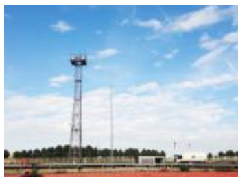
HIGH MAST LIGHT
